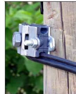
Securing with one bolt
